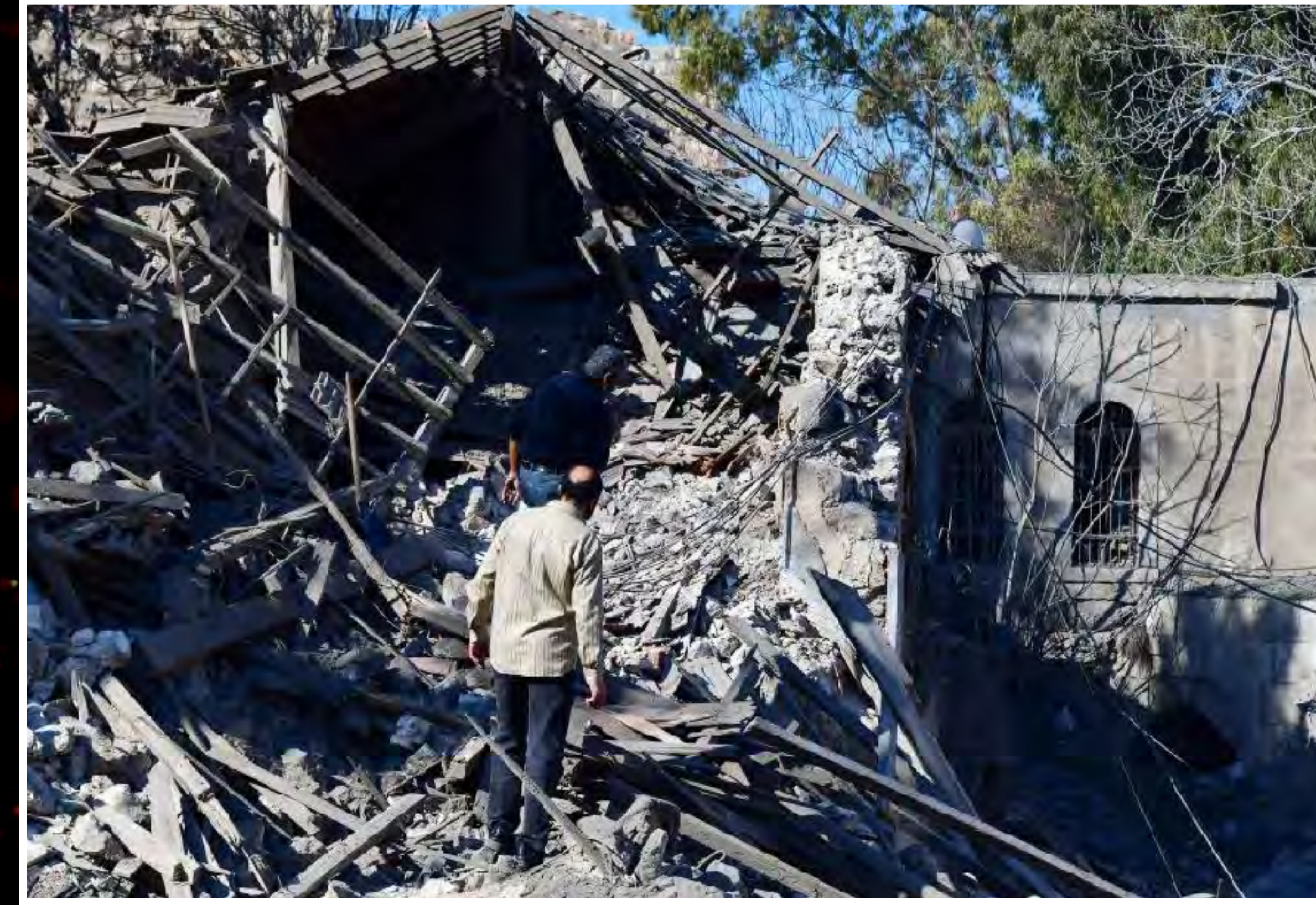
A MAN CHECKS THE DAMAGE FROM AN ISRAELI MISSILE ATTACK INSIDE THE HISTORIC CITADEL IN DAMASCUS, SYRIA, ON FEB. 20.
