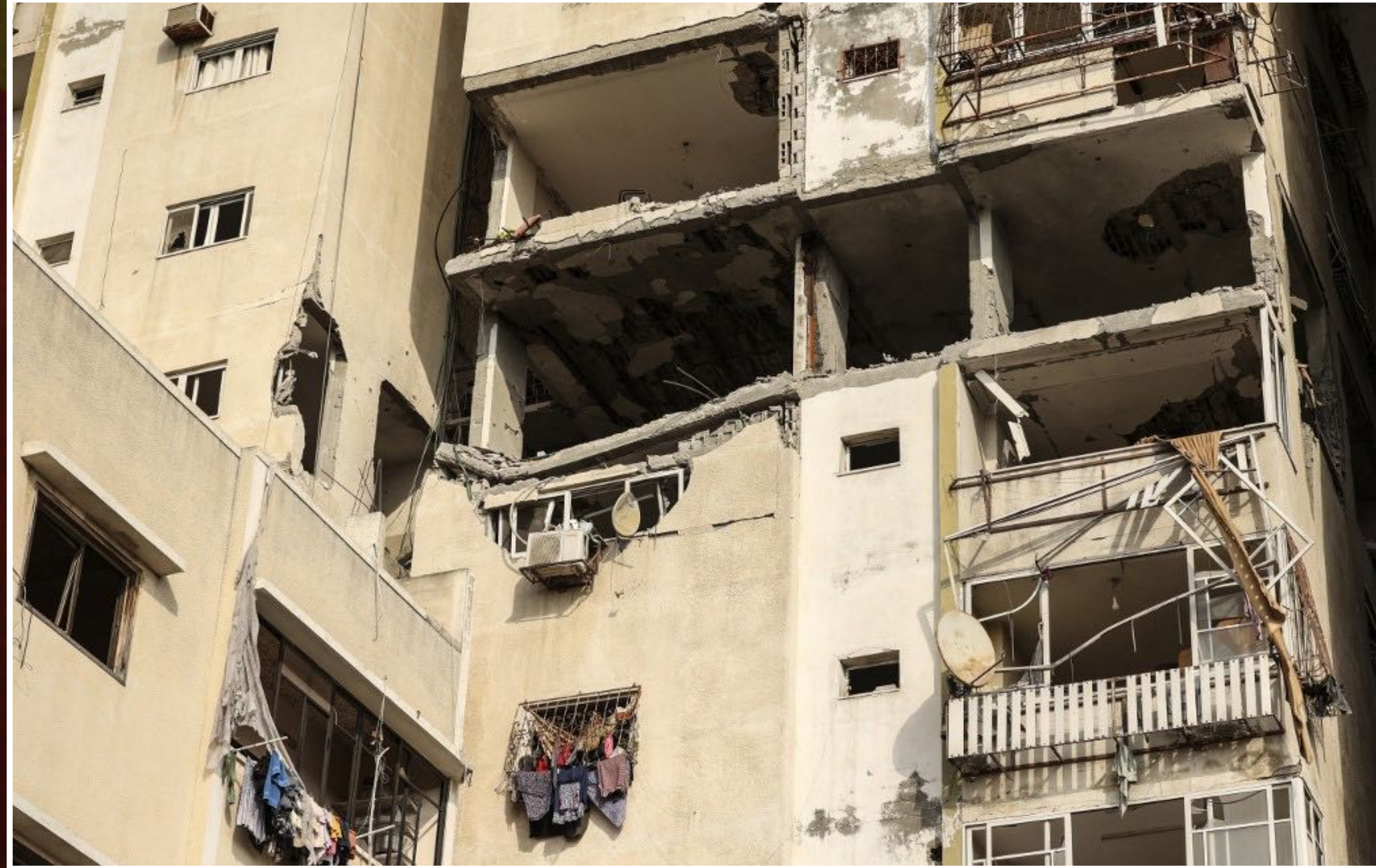
THIS PICTURE SHOWS THE DAMAGE CAUSED BY AN ISRAELI AIR STRIKE ON A BUILDING IN GAZA CITY, ON AUGUST 5, 2022
