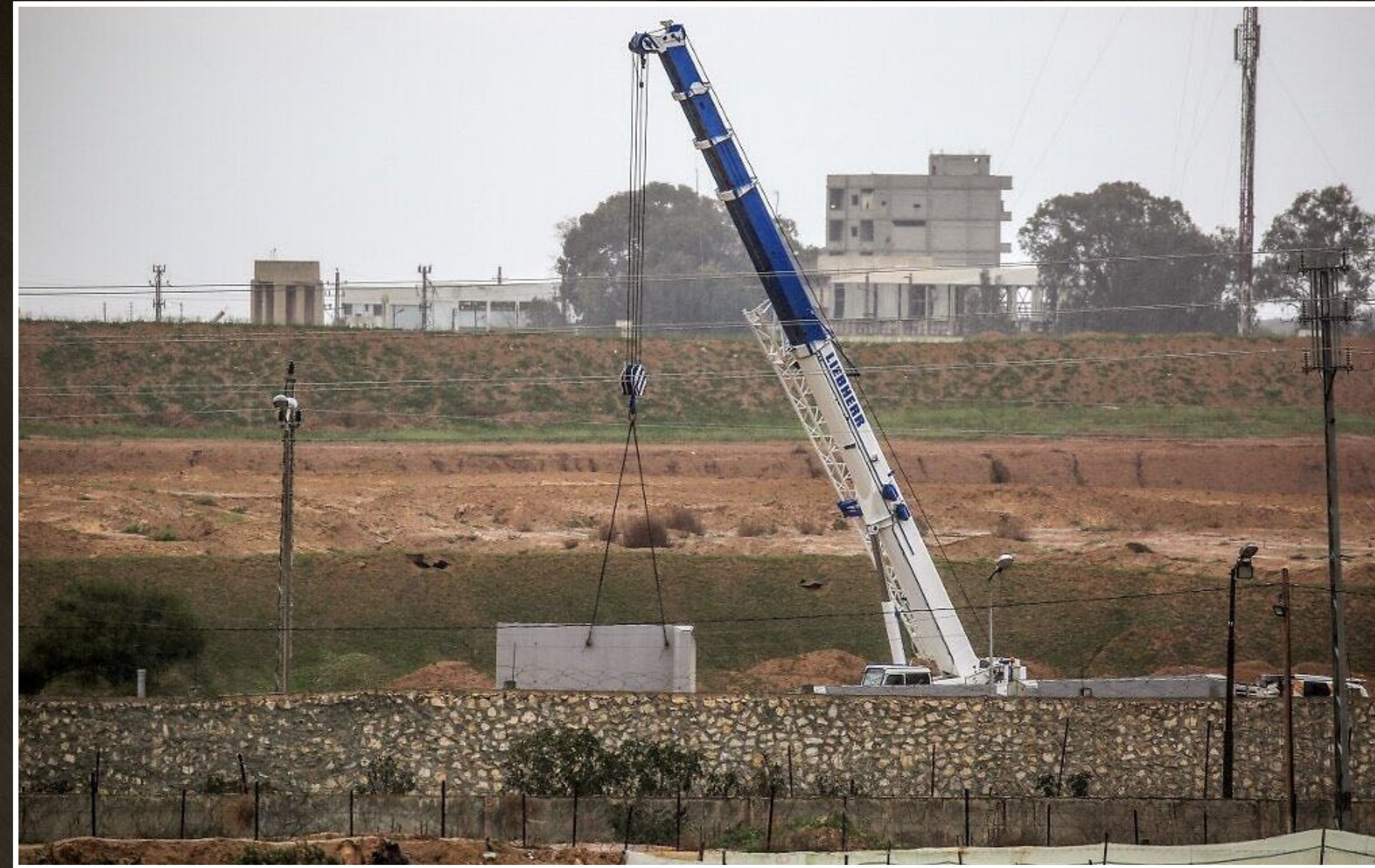
A PICTURE TAKEN IN RAFAH IN THE SOUTHERN GAZA STRIP AT THE BORDER WITH EGYPT SHOWS A CRANE AT THE CONSTRUCTION SITE OF A WALL ON THE EGYPTIAN SIDE OF THE BORDER.
