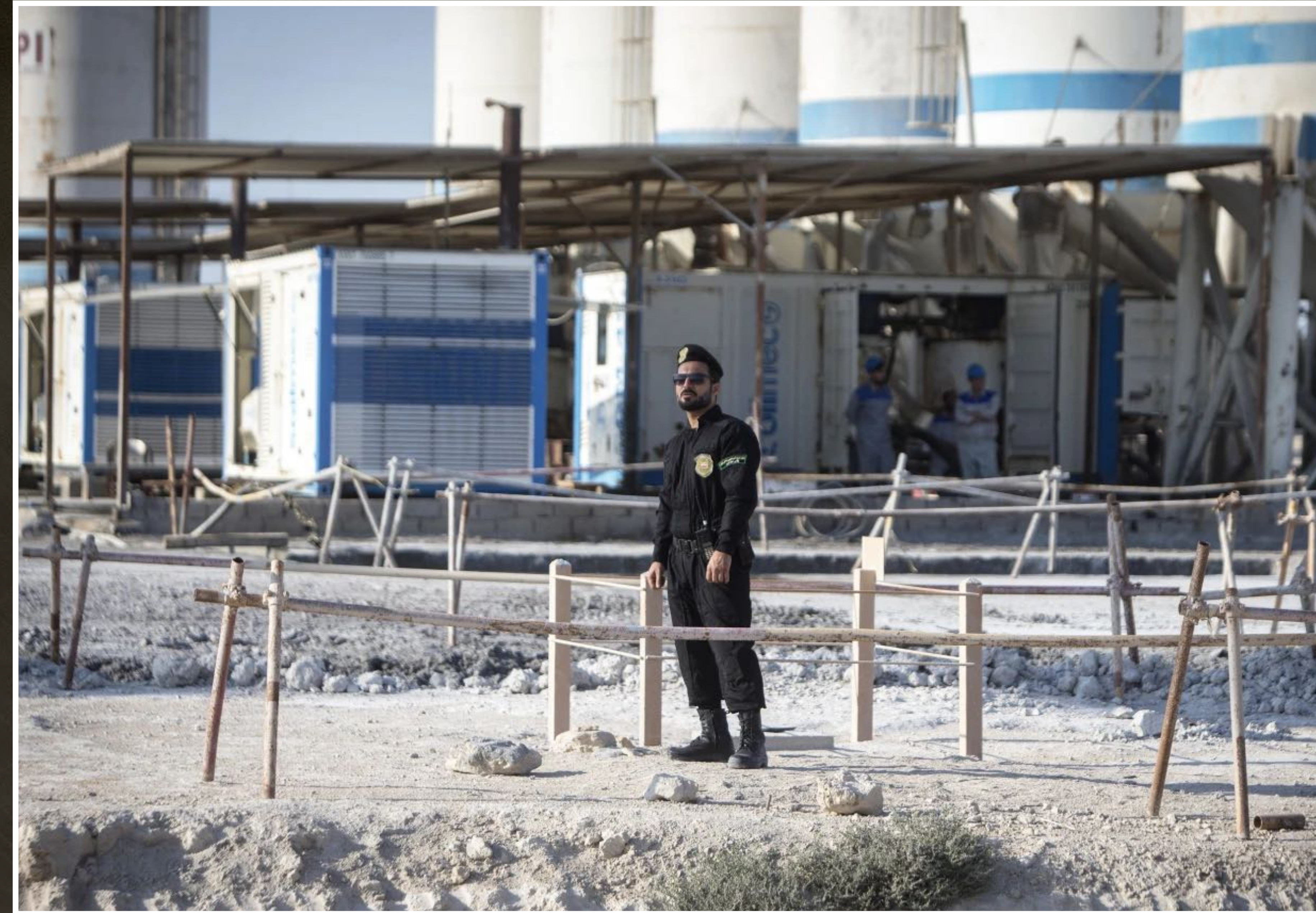
A SECURITY FORCE MEMBER STANDS GUARD AT THE CONSTRUCTION SITE OF THE SECOND PHASE OF IRAN'S BUSHEHR NUCLEAR POWER PLANT
